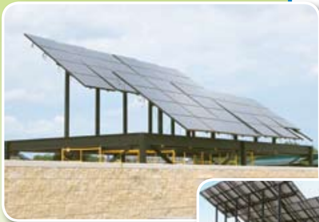
Photovoltaic (PV) cells, seen mounted in solar panel arrays outside NMC's M-TEC building, convert sunlight directly into electricity. When sunlight strikes a PV cell, electrons are dislodged, creating an electrical current.
